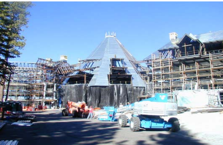
WING B: West side of Head House roof decking is installed
