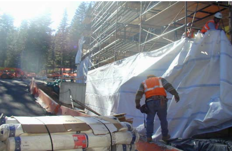
Exterior winterization tenting starts on Wing D
