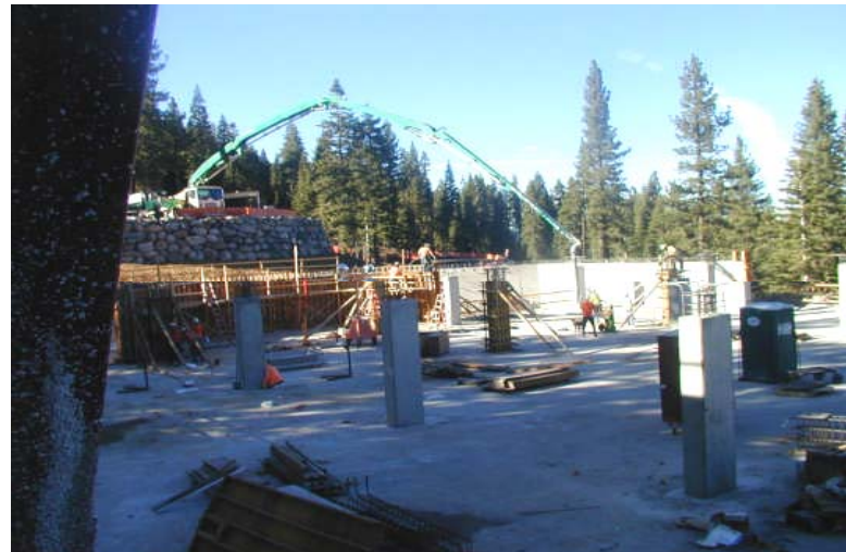
Wall forming on the ramp continues
